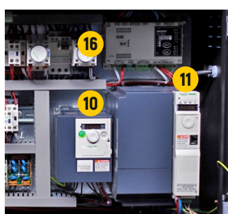
17 / Hoist electric cabinet
