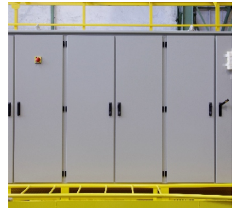
9 / Crane control panel
